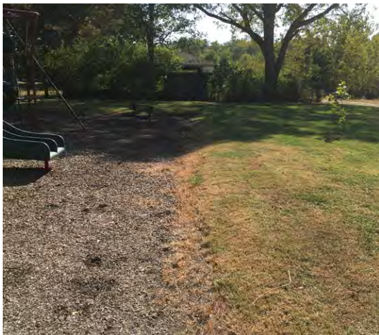
Figure 3.16: The playground safety surface mulch lacks a containment border.
