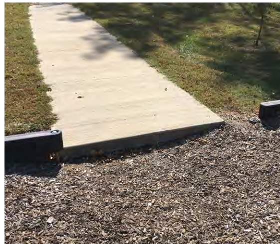
Figure 3.13: Playground safety surface mulch is not level with concrete entry walkway, making it not ADA accessible and creating a tripping hazard.
