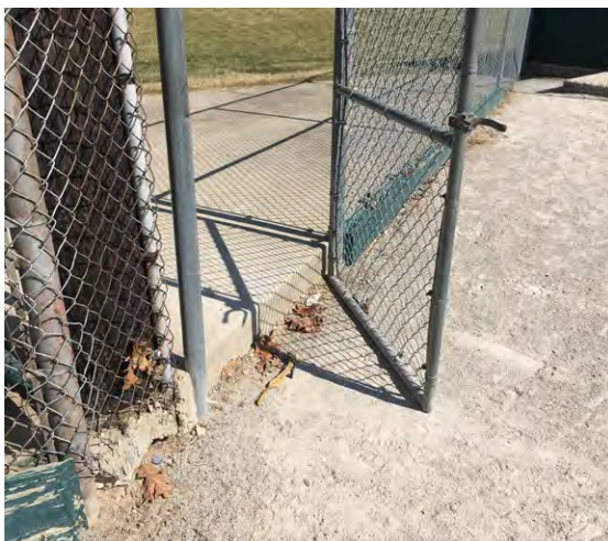
Figure 3.10: The ballfield is not ADA accessible because of a curb at the entrance.
